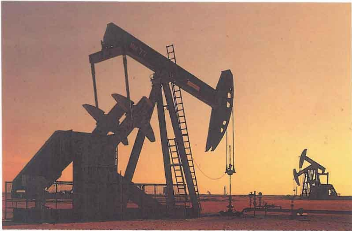
▲ Beam pumps at work in the Nimr oil field, South of Oman.
