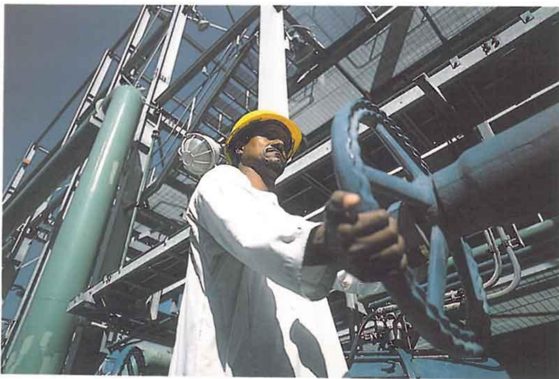
▲ A technician operates machinery at the Al Ghubrah desalination plant which provides water and electricity to the Capital area.
