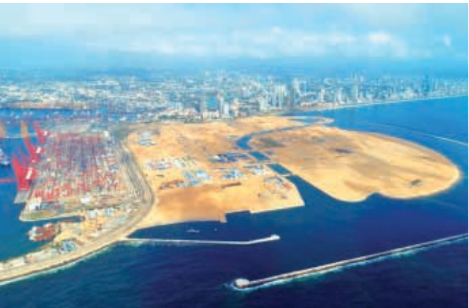
An aerial photo shows a view of the construction site of the Colombo Port City in Colombo, Sri Lanka (Xinhua)
