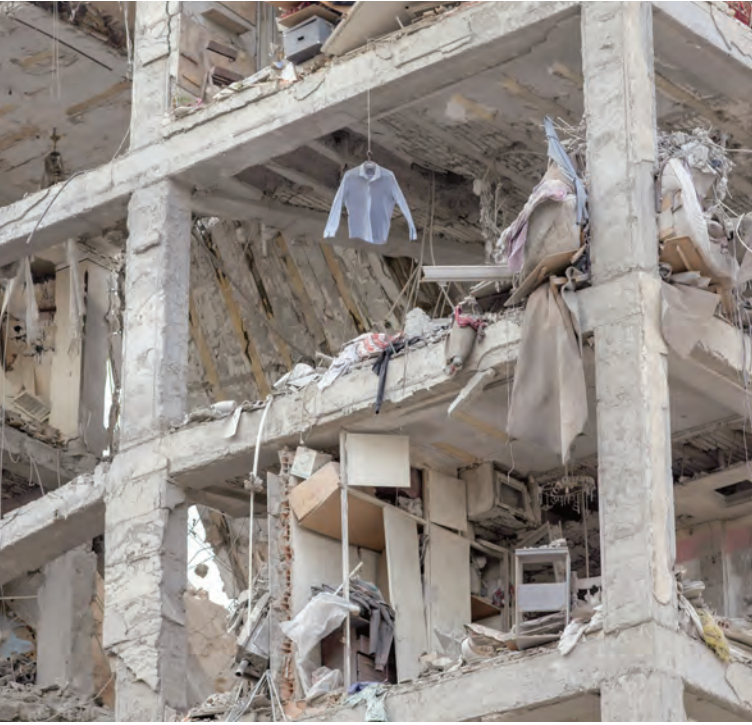
An apartment building damaged in a missile strike in Tehran. — TNYT
