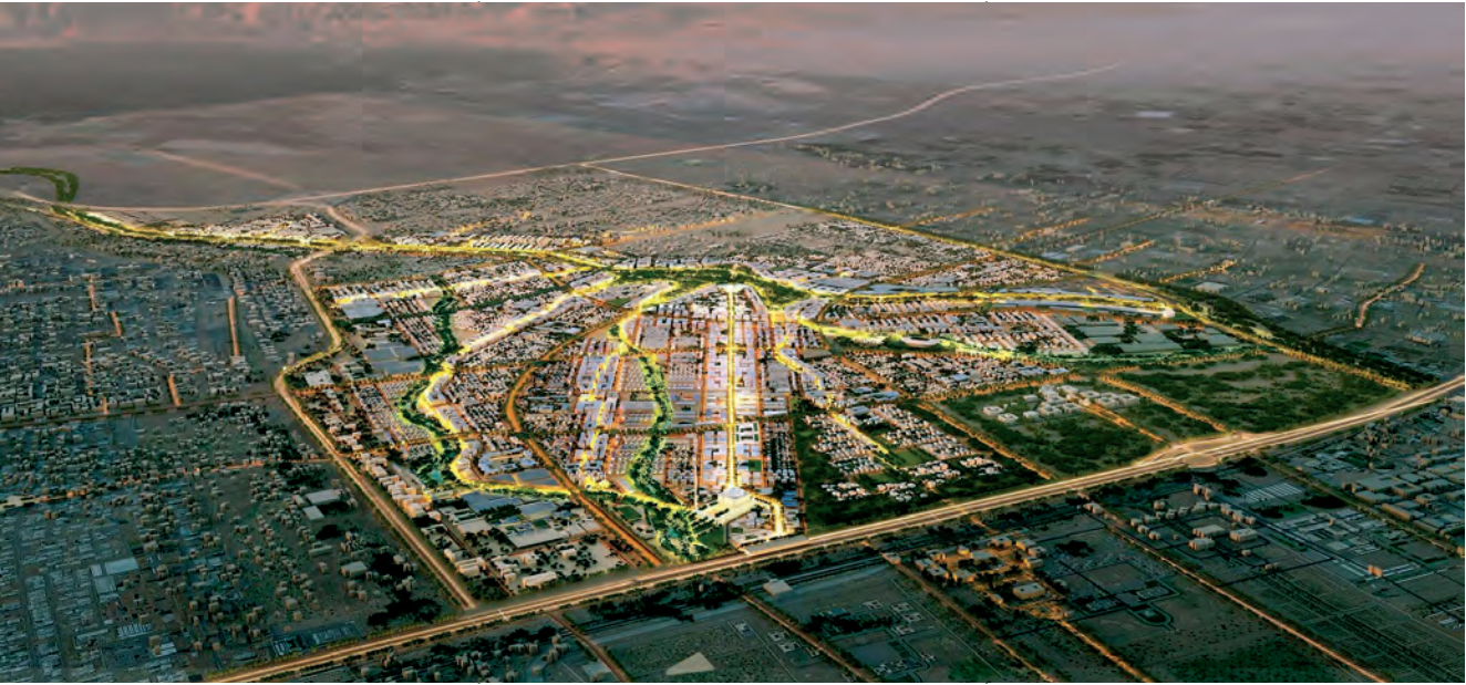
70% of tenders in Phases 1 and 2 of Sultan Haitham City are under execution, with roads and services being rolled out progressively: Dr Al Shueili
