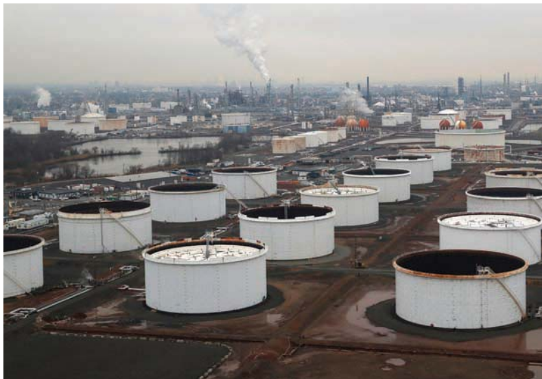
The general view of oil tanks and the Bayway Refinery of Phillips 66 is pictured in Linden, New Jersey, in this file photo. — Reuters
