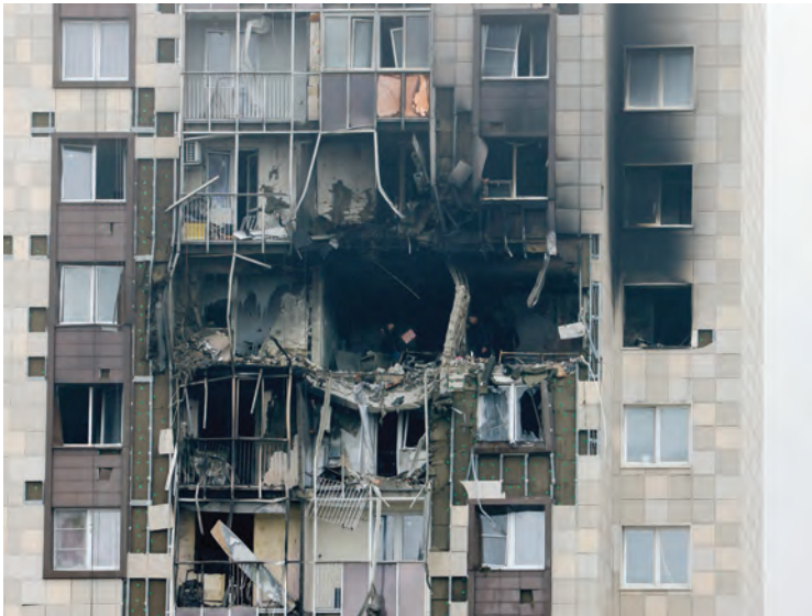
Emergency services personnel work in a damaged multi-storey residential building hit by a Ukrainian drone strike in Kotelniki in the Moscow region. — Reuters
