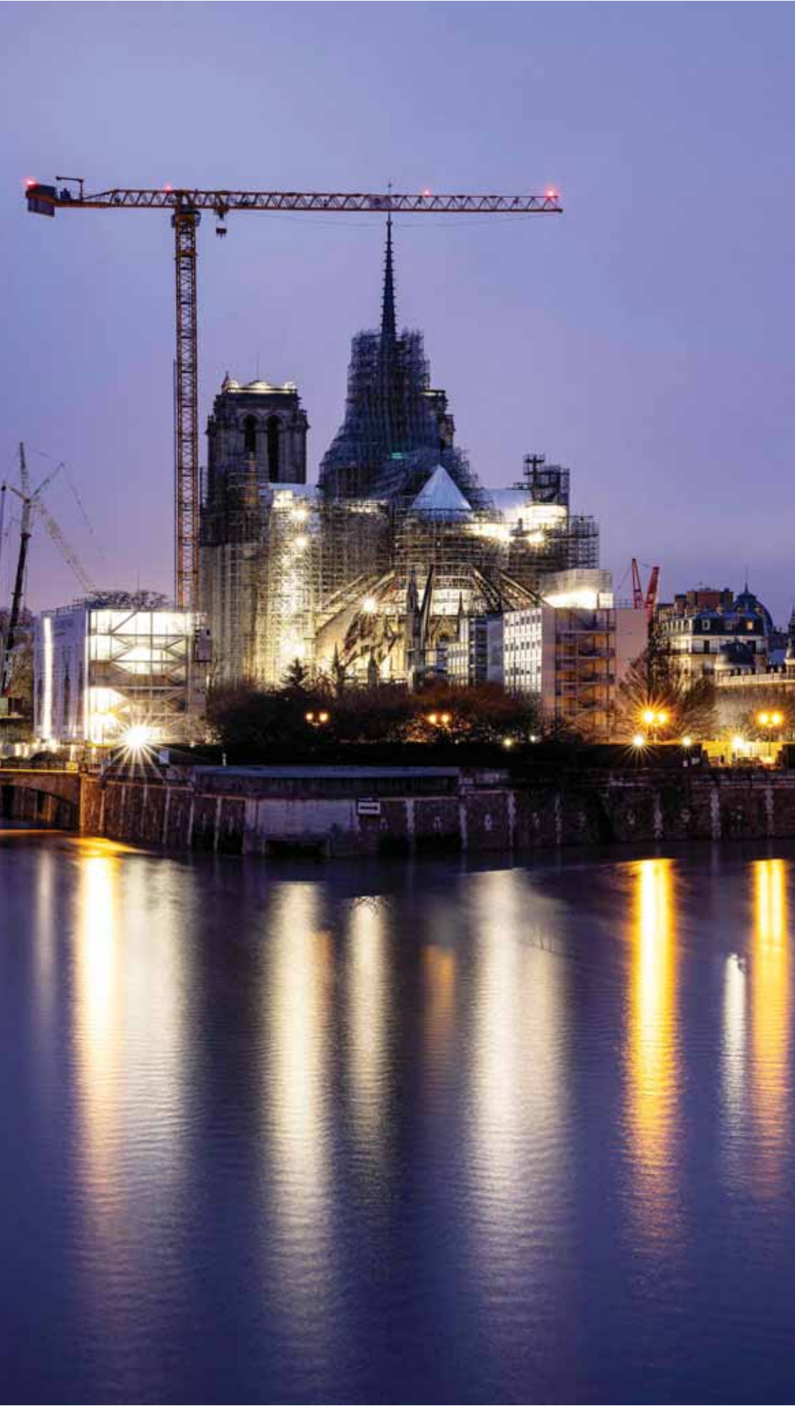
This photograph taken on Sunday shows the construction site of Notre-Dame de Paris Cathedral with its new spire, on Île de la Cité, in Paris. Listed as World Heritage site by Unesco, the 14th century Gothic Notre-Dame Cathedral was partially destroyed including its spire during a fire on April 15, 2019. – AFP
