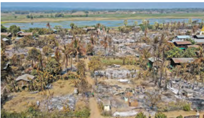
An aerial view of burnt buildings from fires in Mingin Township, in Sagaing Division, on Thursday (AFP)
