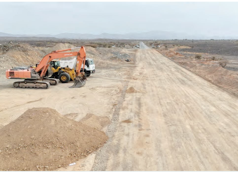
The projects form part of the 2025 road paving plan for Al Sharqiyah North Governorate.
