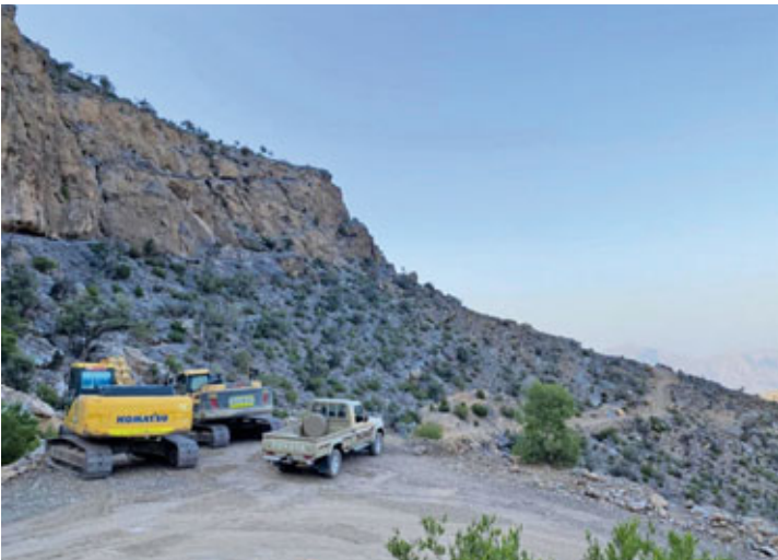
COMMUNITY INITIATIVE: The two-phase project to reconstruct and rehabilitate the mountain road is a community initiative.
