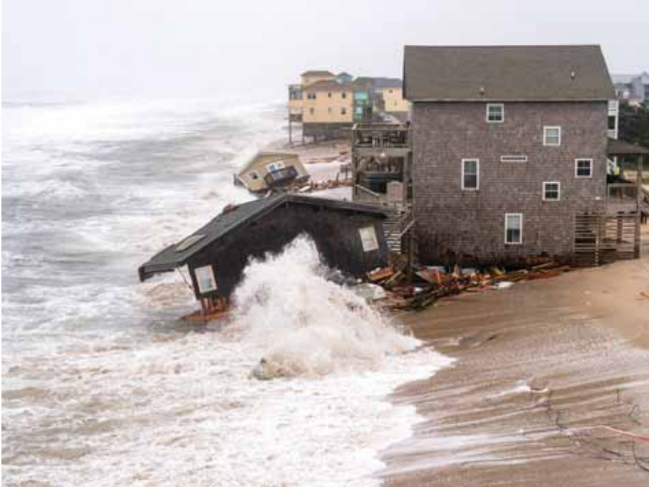
Two homes collapse into the Atlantic Ocean on the coast of Rodanthe, NC, after a storm.
