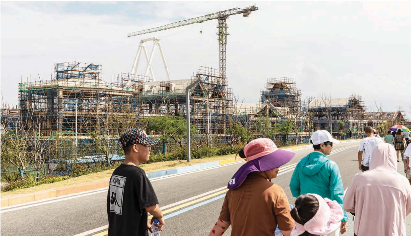
Discontinued construction is seen at an amusement park in Nantong, China. — The New York Times
