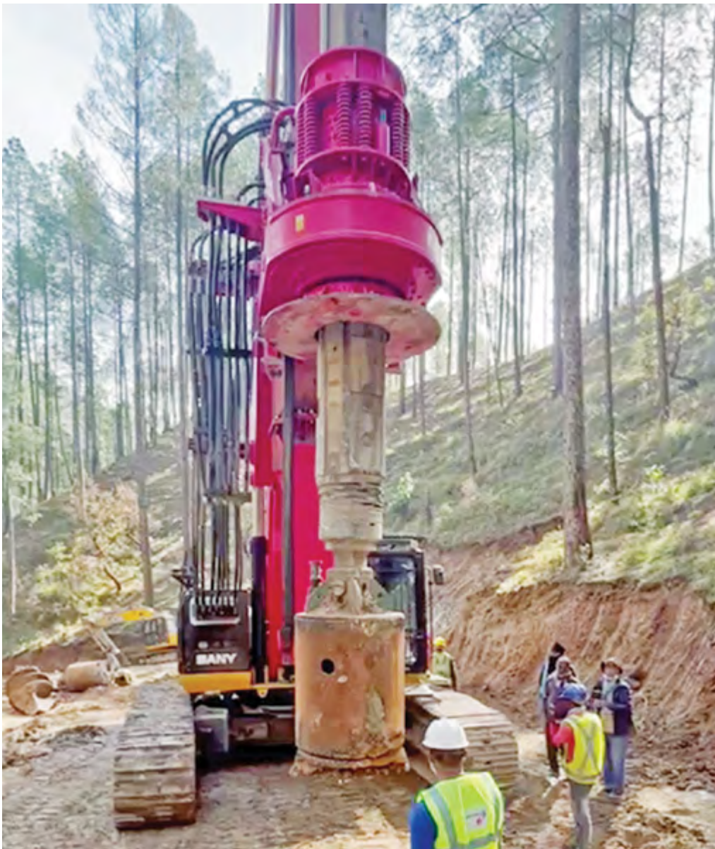
SJVN begins vertical drilling work on the top of the Silkyara tunnel, in Uttarkashi, India, on Sunday (ANI)
