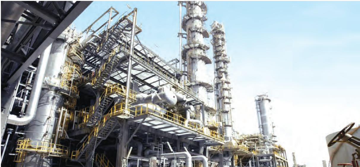
The project will be established at dual locations within SOHAR Port and Freezone (Picture for illustration).
