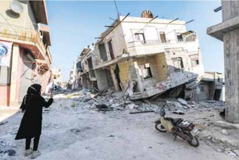
Collapsed buildings are seen along an alley in the aftermath of the February 6 deadly earthquake that hit Syria and Turkiye, in Jindayris, northwestern Syria. — AFP
