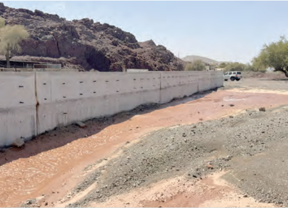
These efforts are part of broader initiatives to mitigate flood risks and safeguard agricultural lands. — ONA
