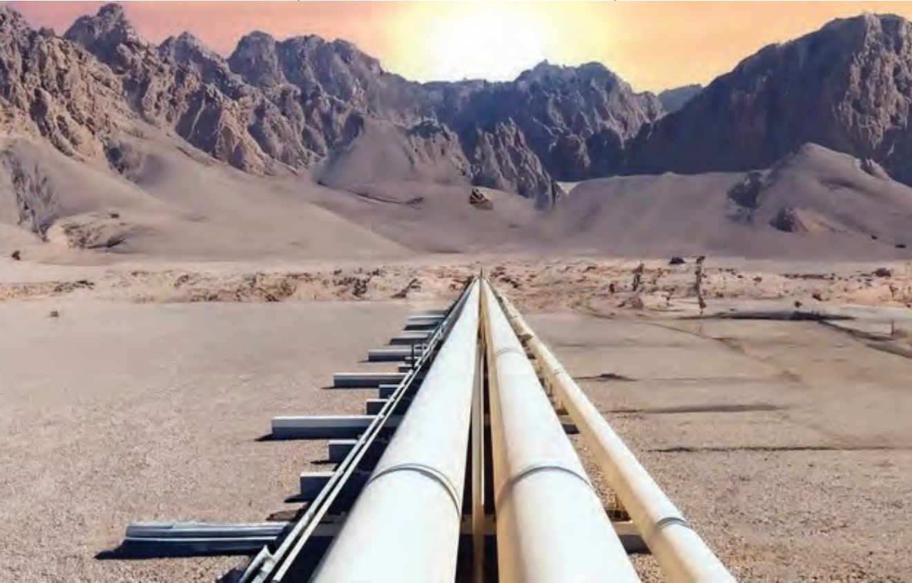
When operational, the projects will contribute to expanding OQGN’s overall pipeline network to 4,717 km by 2027
