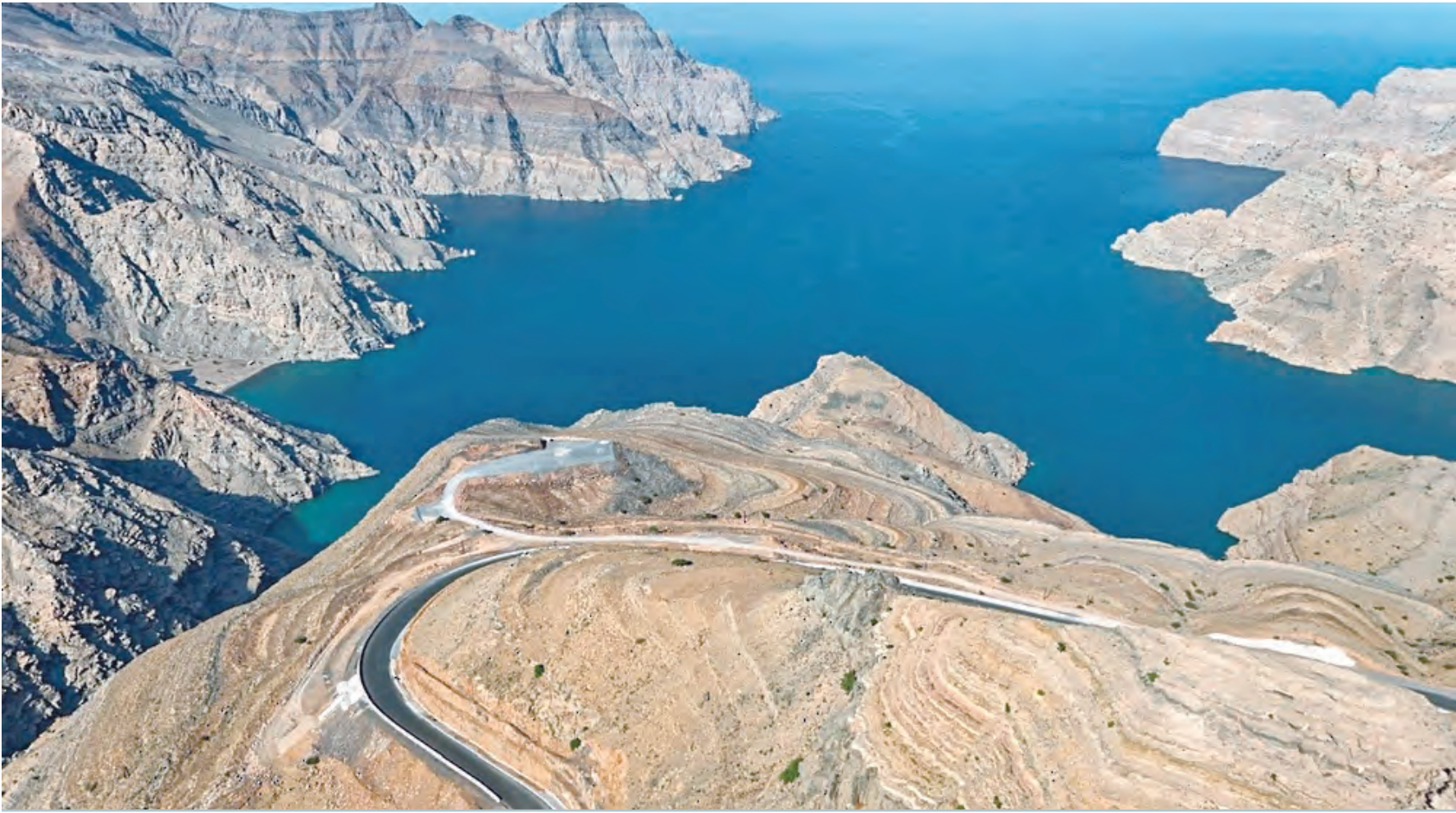
The completion rate of the Sultan Faisal bin Turki Road project (Dibba-Lima-Khasab) in the Governorate of Musandam has reached approximately 76 per cent. The project, valued at RO 151 million, being executed by the Ministry of Transport, Communications and Information Technology, is among the strategic infrastructure initiatives aimed at enhancing the road network and strengthening connectivity between the governorate's wilayats. DETAILS ON P2
