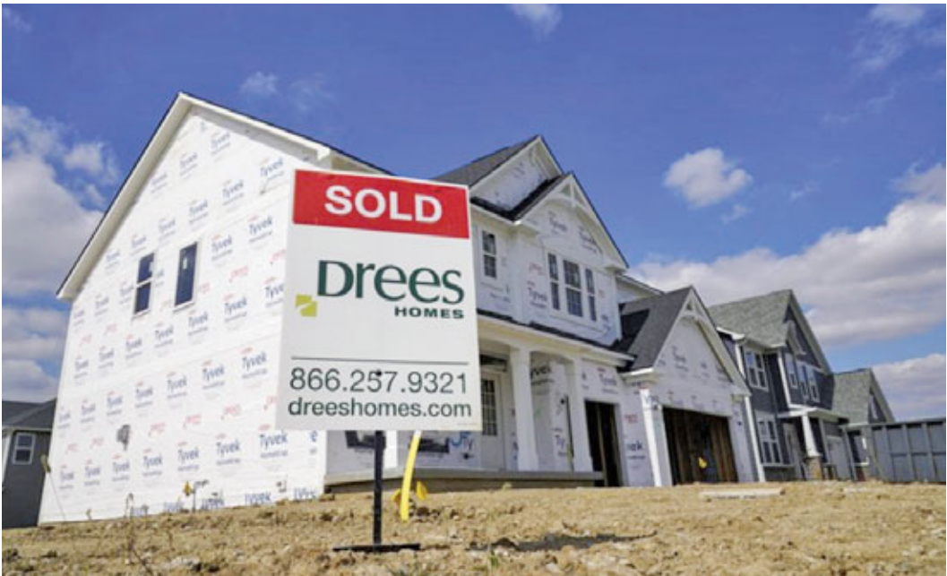
REPORT: According to the report, applications for building permits, a good sign of future activity, increased by 2.7 per cent to a seasonally adjusted annual rate of 1.77 million units. - BNA
