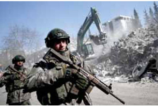
Turkish soldiers patrol next to collapsed buildings in Kahramanmaras. – AFP
