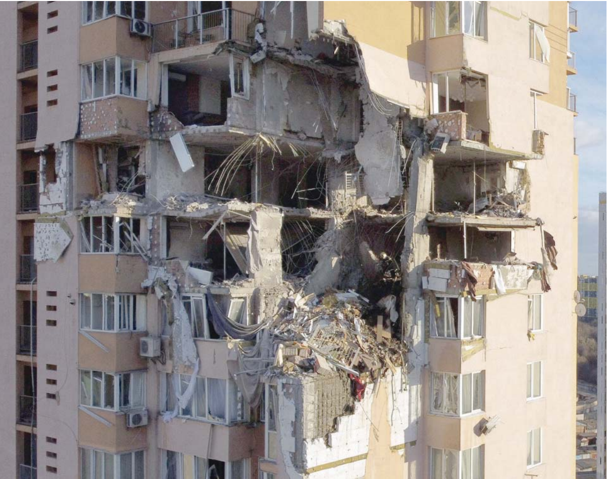
A general view shows damage to the upper floors of a building in Kyiv after it was reportedly struck by a Russian rocket. — AFP
