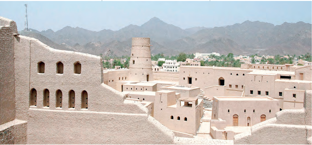
The “Revival of Earthen Architecture” initiative focuses on reintroducing clay using modern engineering methods that aim to improve performance while maintaining its cultural and environmental value.
