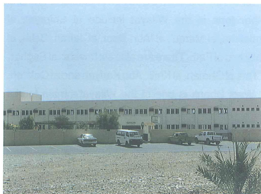
Education is provided in modern buildings
