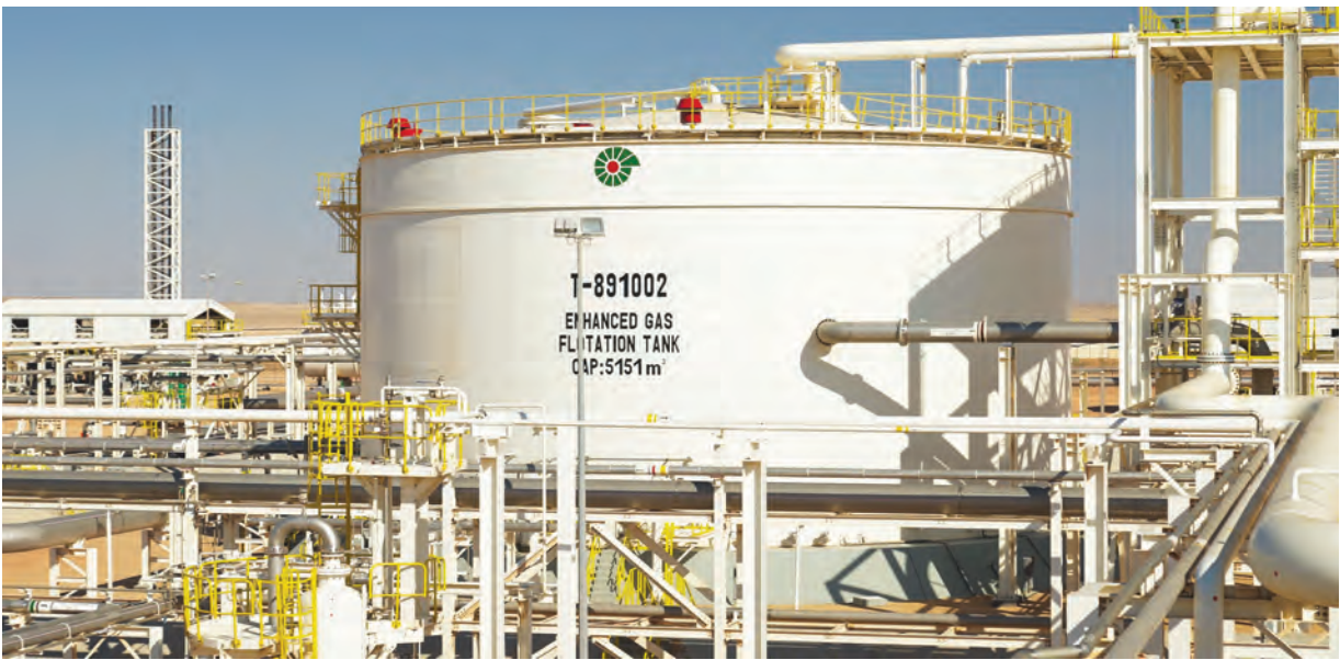
Gas revenue slumped 38% in Q1 2024.
