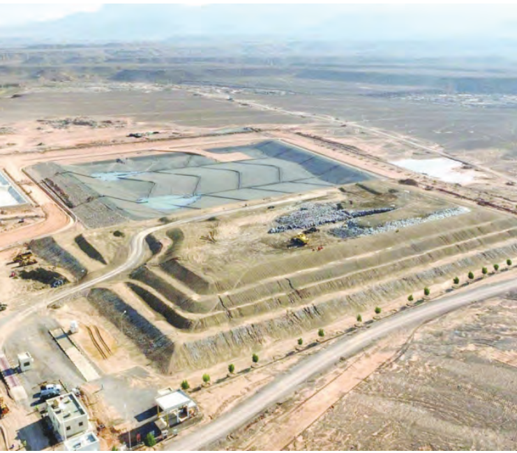
The largest completed expansion was at Tahwa Landfill, where a new engineered cell added 1.9 million tonnes of disposal capacity.
