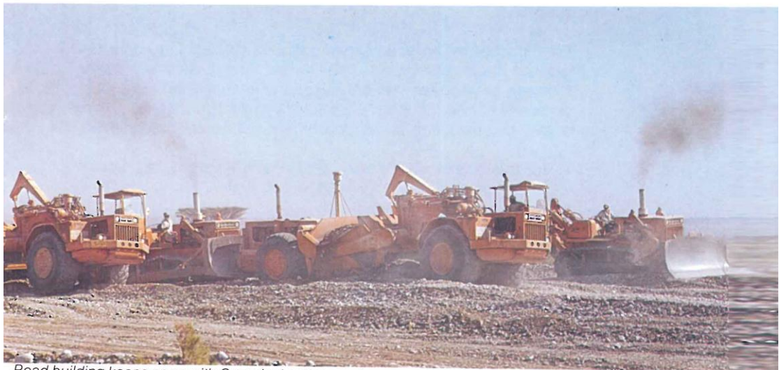
Road building keeps pace with Oman's development.
