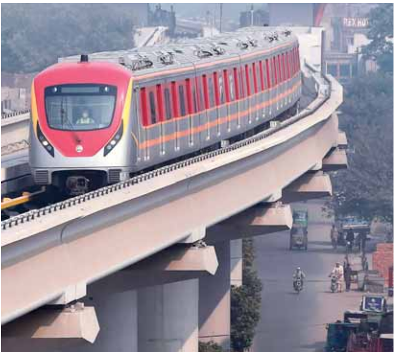
Pakistan's first-ever metro train service, the Orange Line, started its commercial operation Sunday in the country's historical city of Lahore opening a new stage for the South Asian country in the public transportation sector. — AFP
