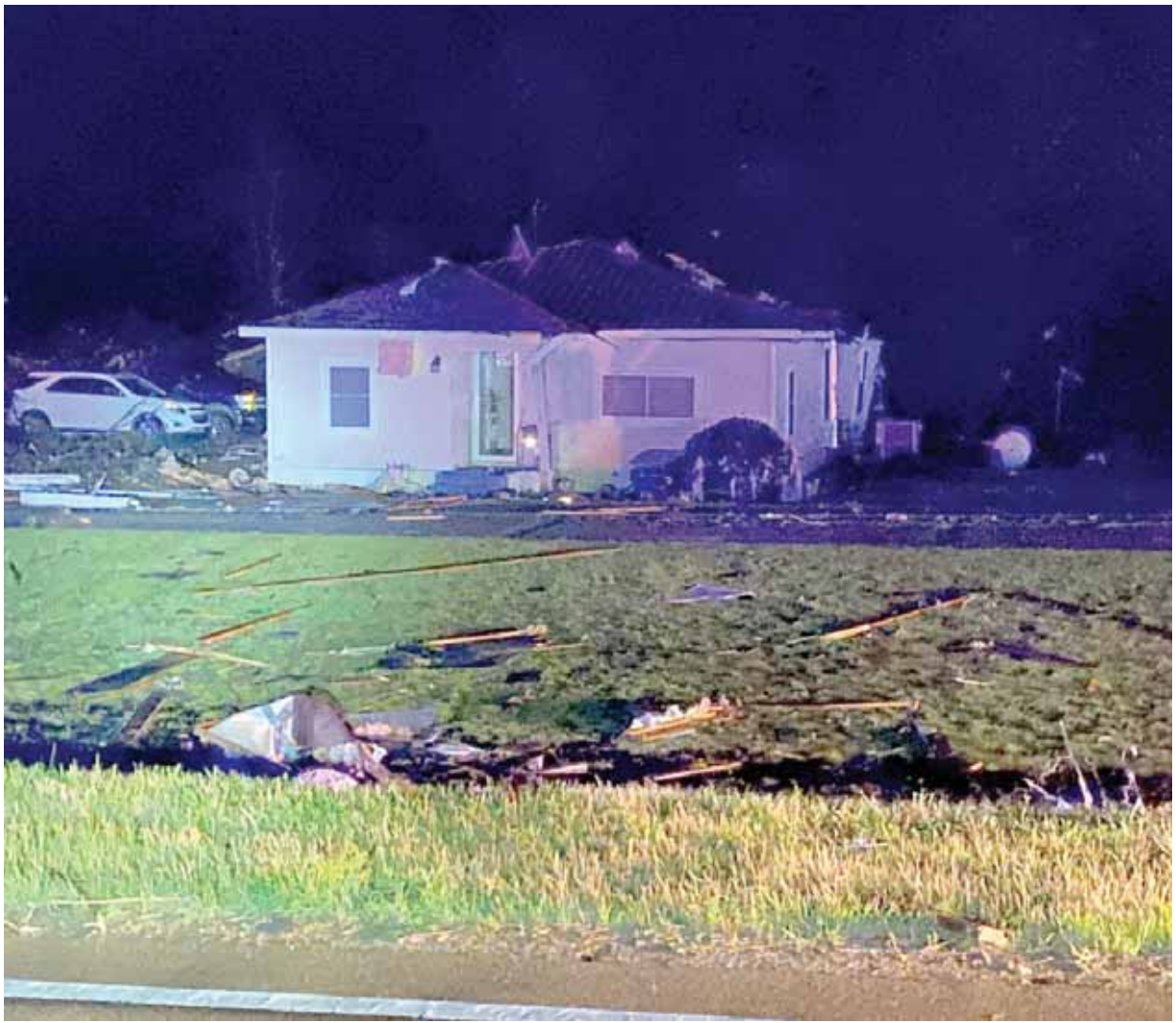
A general view shows a damaged building, following a tornado in Silver City, Mississippi, US, on Saturday. — Reuters
