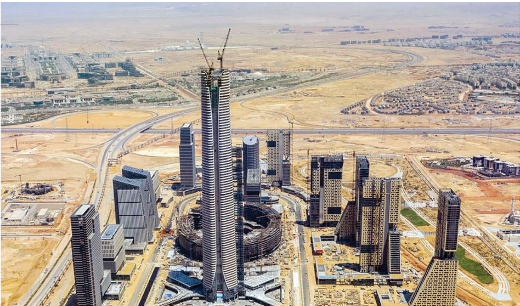
CBD project in Egyptian capital boosts local development Aerial picture shows the Central Business District (CBD) project in Egypt's new administrative capital in east of Cairo, Egypt. The construction of the CBD in Egypt's new administrative capital has injected new vitality into the country's economic and social development. Xinhua
