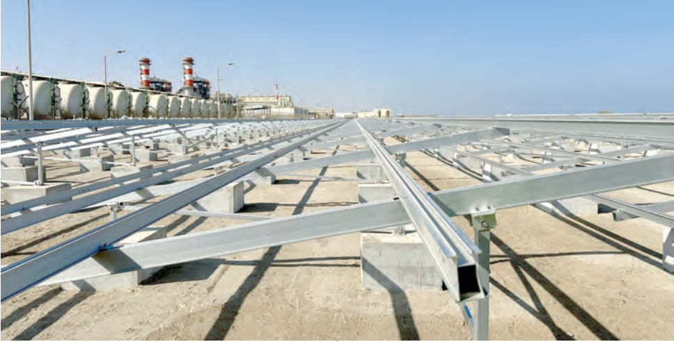
Solar farm under construction adjacent to the Barka V IWP.
