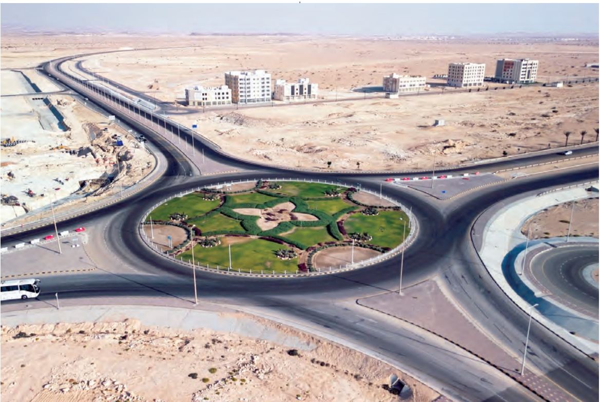
The dualiation of the Sultan Said bin Taimur Road (National Road 32/South) aims to improve traffic in the centre of Duqm city.
