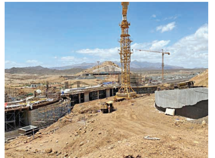
Construction work of the sultanate's first cable car in progress at Oman Botanic Garden in Al Khoudh, Seeb (Supplied photo)
