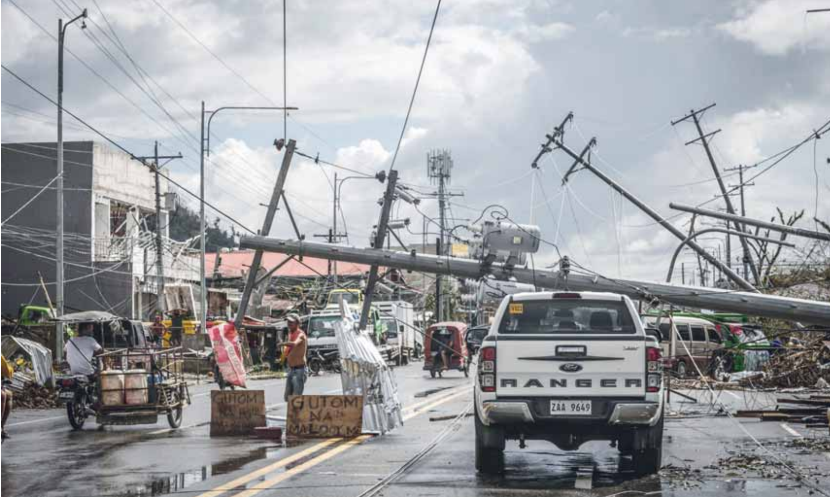
Fallen electric pylons block a road in Surigao City days after super typhoon Rai devastated the city. — AFP
