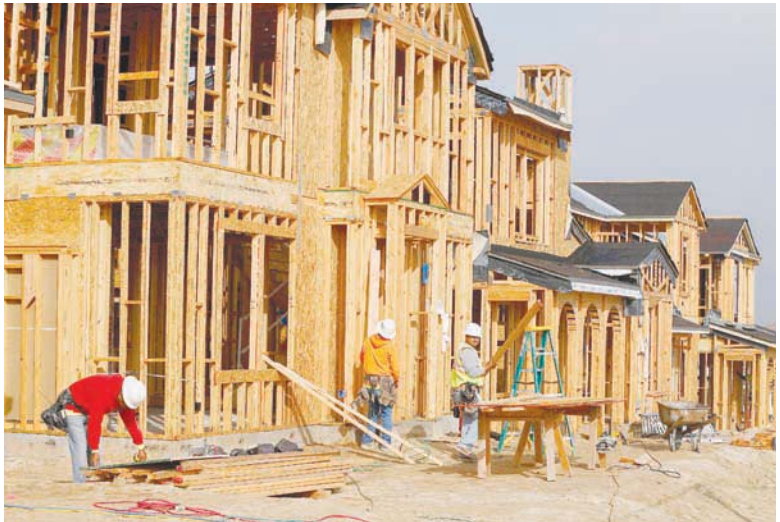
Construction workers build single homes in San Diego, California. — Reuters
