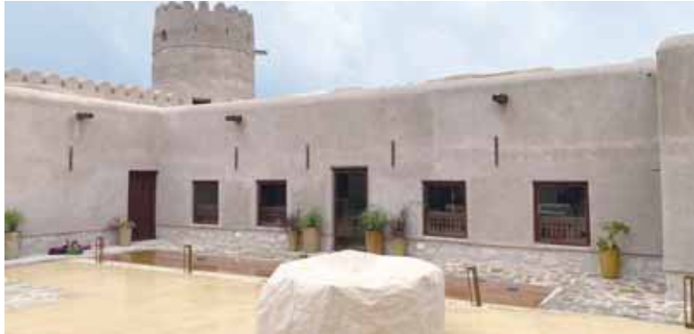
The Al Khamis Wall and Tower in Al Musannah
