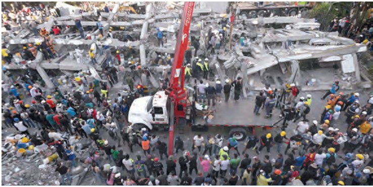
Rescuers and volunteers search for survivors amid the rubble of a collapsed building after an earthquake in Cali, Colombia. — AFP
