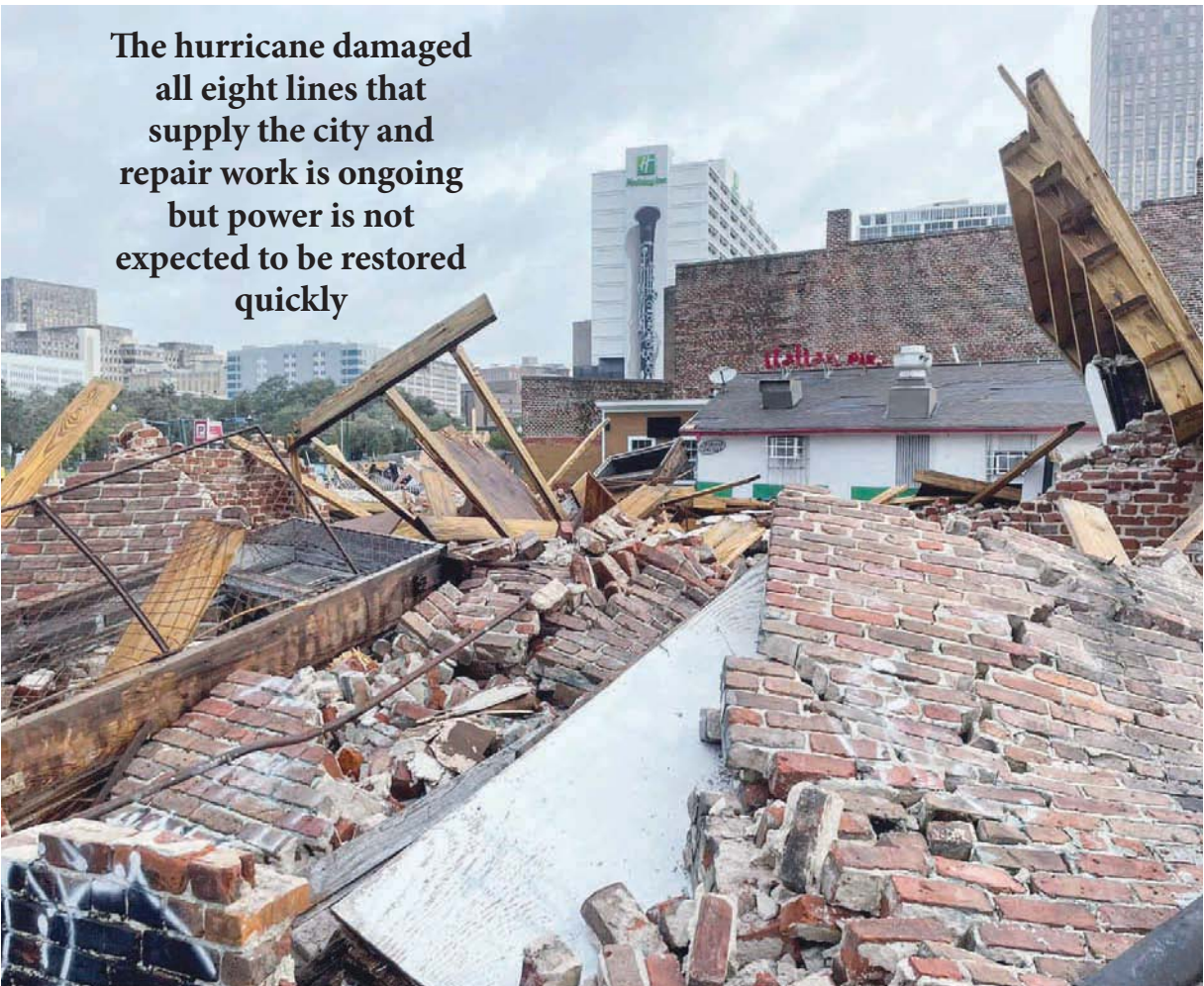
The Karofsky shop suffers severe damage after Hurricane Ida pummelled New Orleans with strong winds in Louisiana. — Reuters
