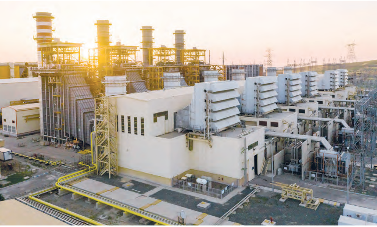
Energoprojekt ENTEL (EPE) announced that it has secured a major consultancy services contract from Nama PWP covering the development and tendering of three CCGT projects.
