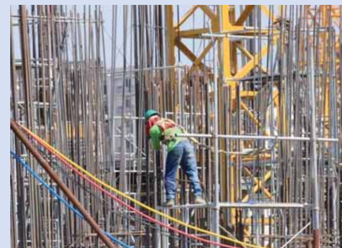
A worker installs steel rods at a construction site in Paranaque city, Metro Manila, Philippines. — Reuters
