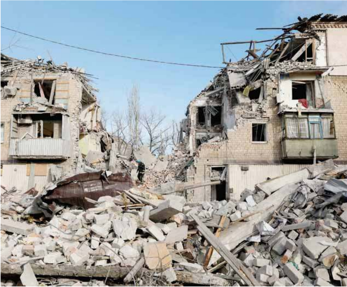
A view shows residential houses heavily damaged by a Russian missile strike, in the town of Selydove, Donetsk region, Ukraine. – Reuters
