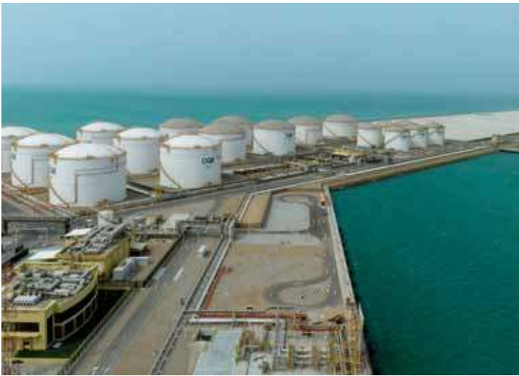
The Ras Markaz Crude Oil Storage project
