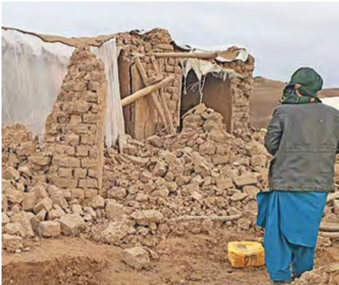
A resident stands near a damaged house at Qadis district in the southern part of Badghis province on Tuesday (AFP)
