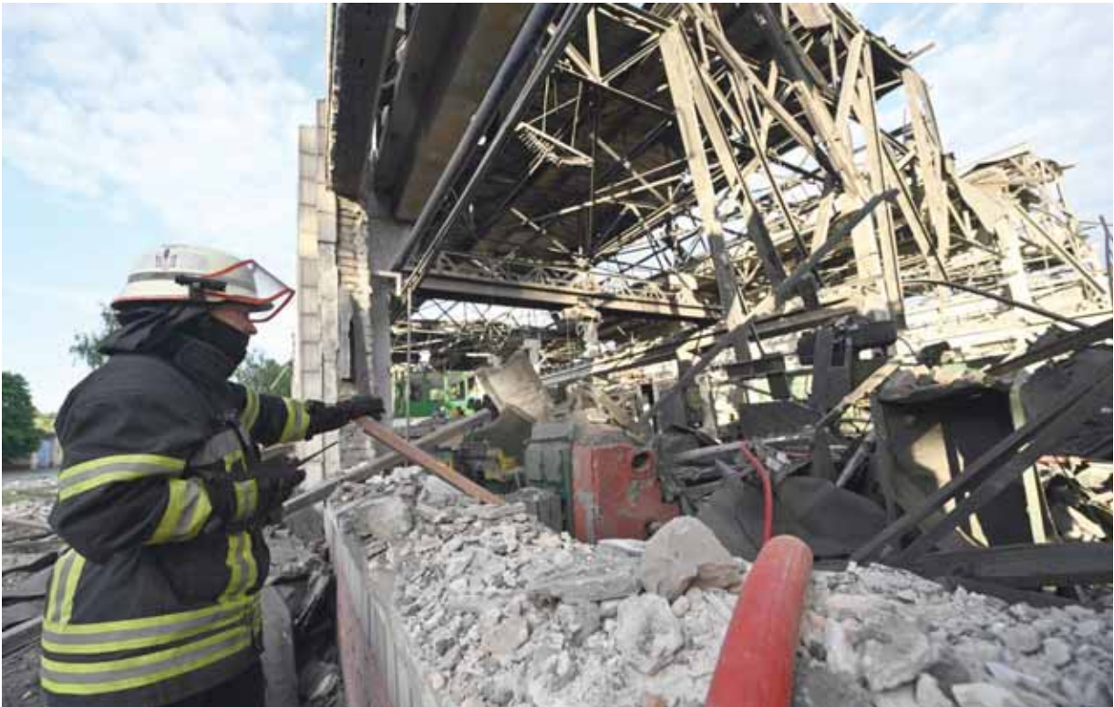
A firefighter stands in a destroyed production depot of the Darnytsia freight cars repair plant, which was targeted by Russian missile strikes in Kyiv. — AFP
