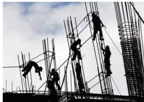
Workers construct beams of a building in Navotas City, Metro Manila. — Reuters
