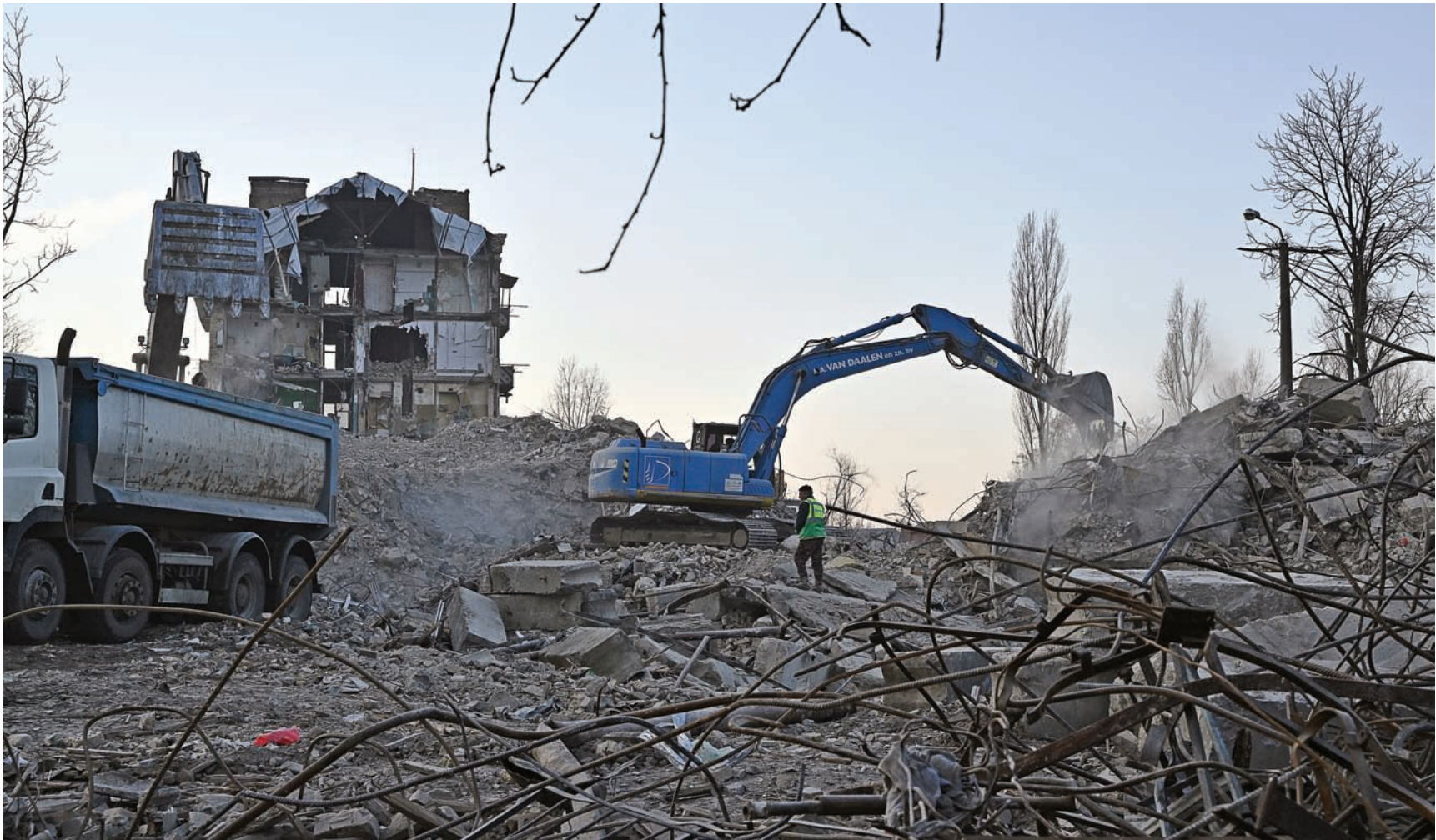
Workers dismantle a heavily damaged residential building in Irpin, northwest of Kyiv, on December 23, amid the Russian invasion of Ukraine (AFP)
