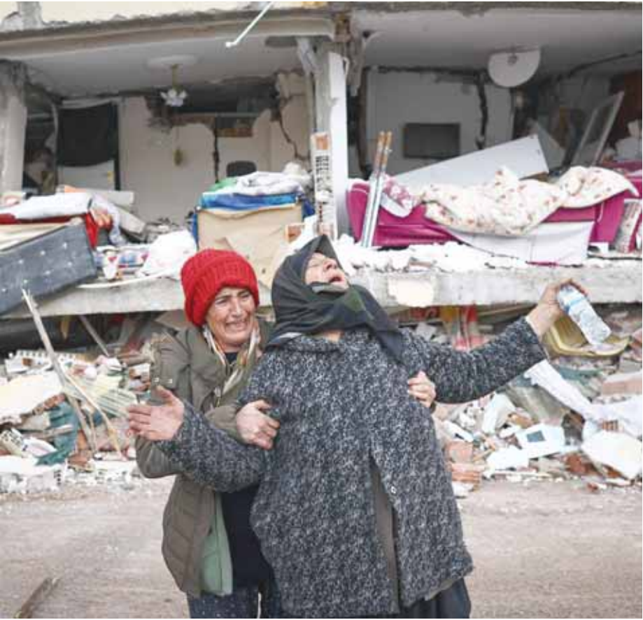
Women react at the site of a collapsed building in the aftermath of the major earthquake in the Elbistan district of Kahramanmaraş, Türkiye, in February.
