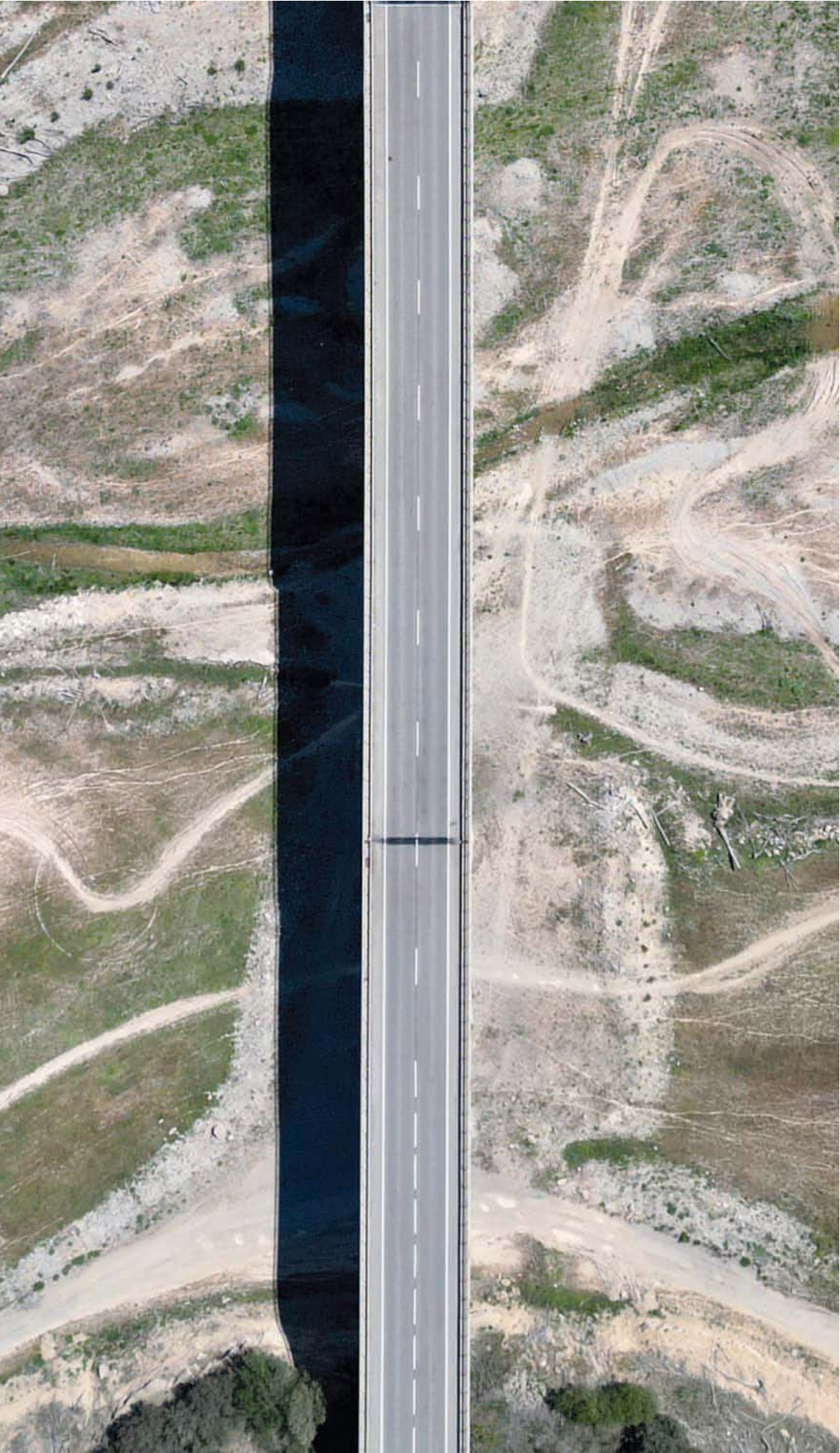
A view shows the cracked ground of the Rialb reservoir as drinking water supplies have plunged to their lowest level since 1990 due to extreme drought, in the village of Bassella, Spain. — Reuters
