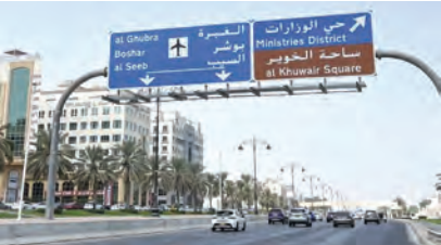
The project has entered the sign manufacturing and physical installation phase.
