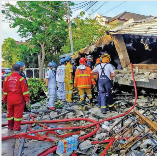
Rescue workers at the wreckage of a collapsed building, in Thailand's capital Bangkok on Saturday (AFP)
