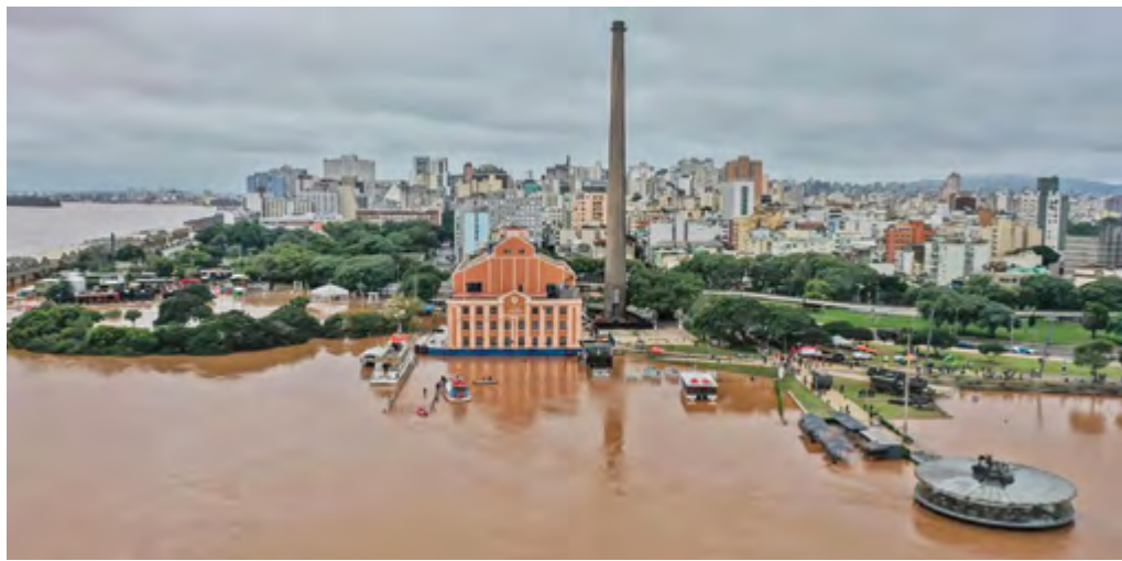
A view of the flooded urban area in Porto Alegre, Rio Grande do Sul, Brazil
