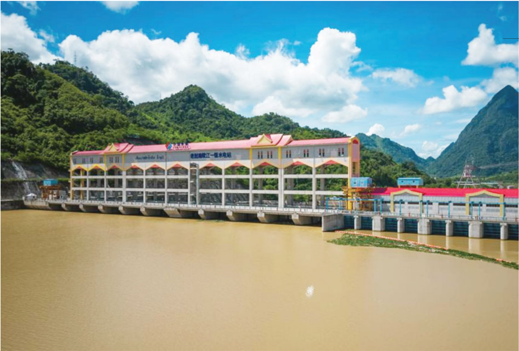
Nam Ou hydropower project in Laos Aerial picture shows the Nam Ou 1 hydropower plant of the Nam Ou River Cascade Hydropower Project in Luang Prabang, Laos. The Nam Ou project includes seven cascade hydropower plants along the Nam Ou river which is the largest tributary of the Mekong river in Laos. Xinhua
