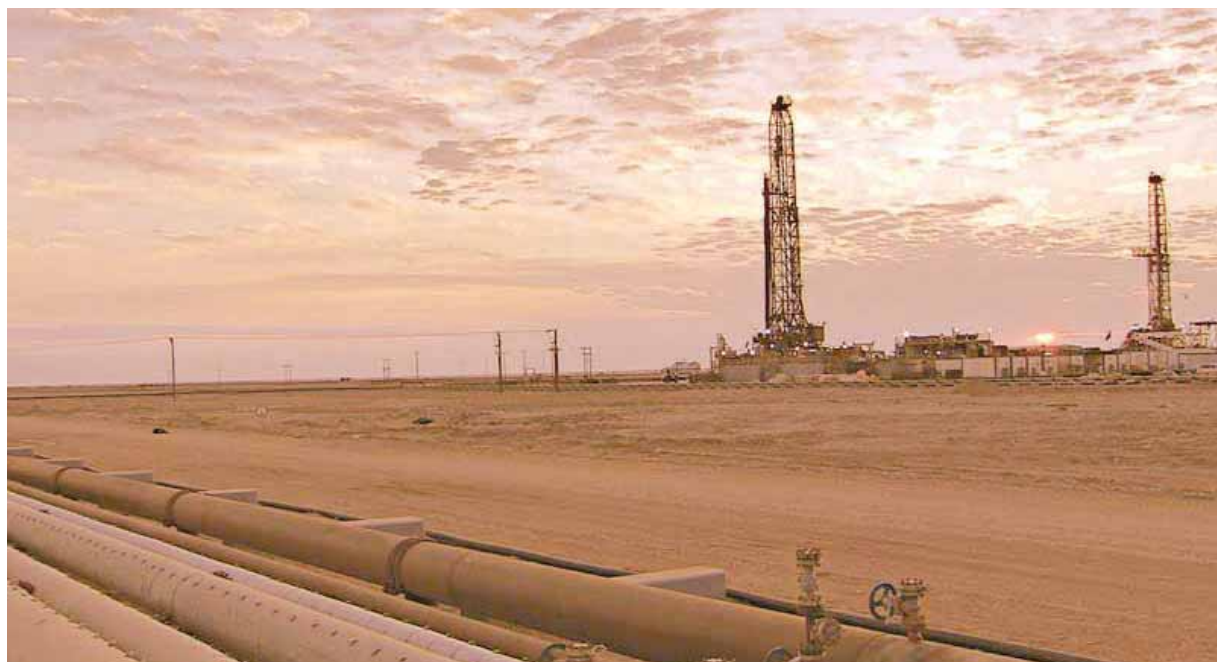
Facilities at Oxy Oman's Mukhaizna field in Block 53.
