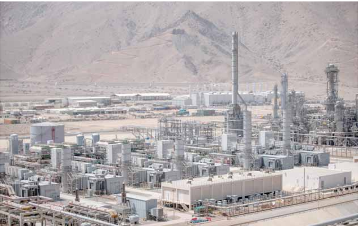
Oman's crude oil and oil condensates reserves stood at approximately 4,971 million barrels. – ONA
