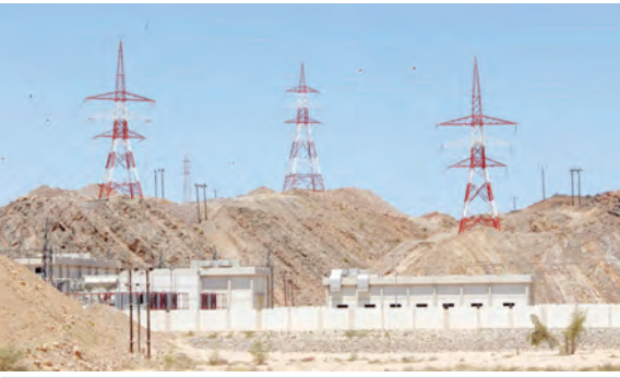
All electricity lines located in wadis have been assessed and are now in the design phase.
