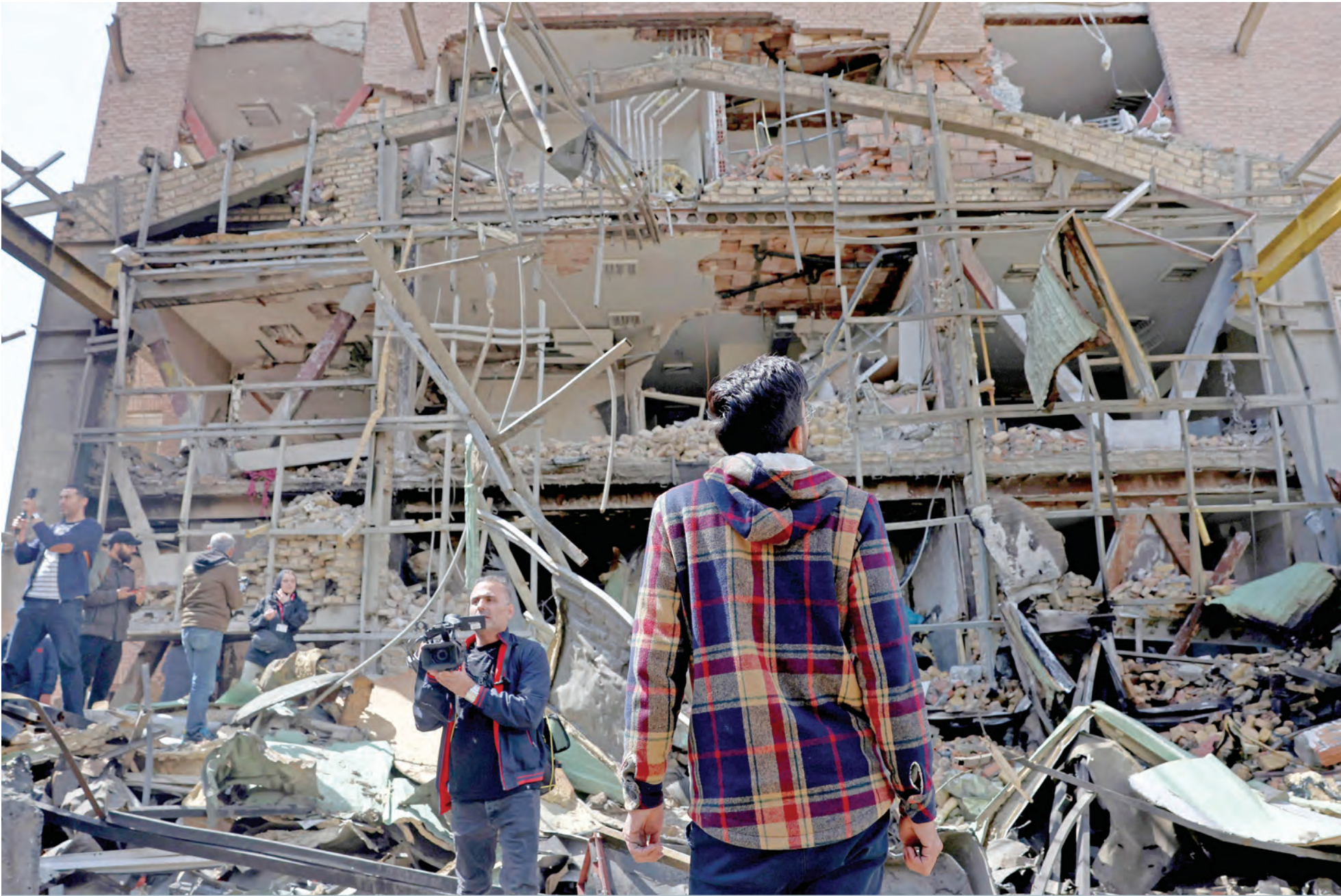
Media representatives gather around the damaged building of the Shahid Beheshti University following a strike, in Tehran. — AFP
